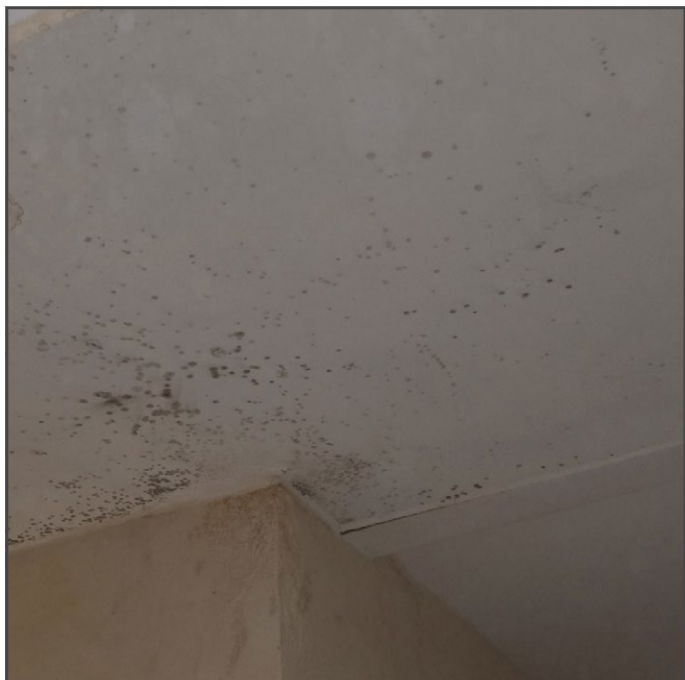
STEP 1 Inspect the property for mould and mildew.
